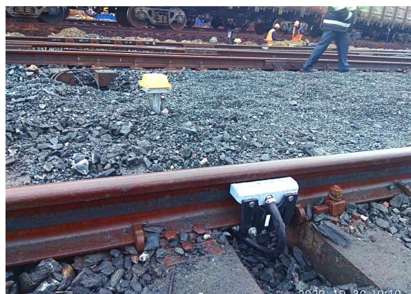
The on-site-installation of the RSR180 is shown on this picture.
